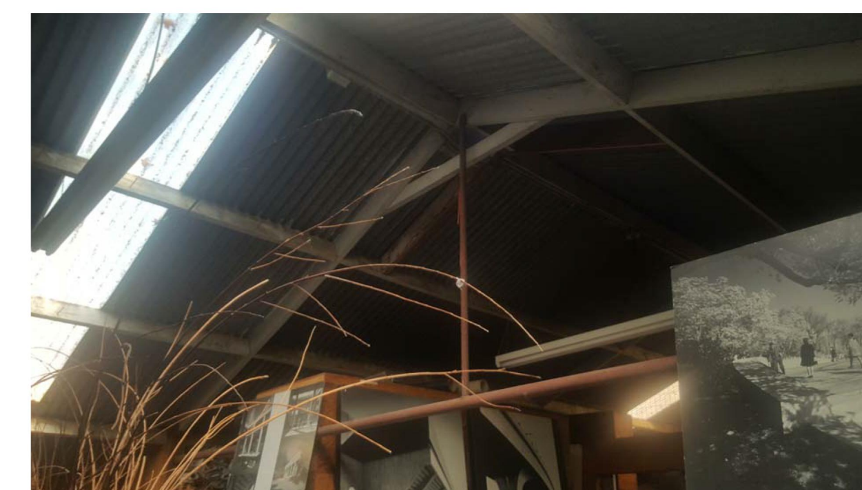
ARCHIVE ROOF TRUSS
